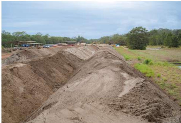
3 Treated soil is moved to lined beds to allow continuous monitoring of hydrocarbon degradation and soil quality improvement.
