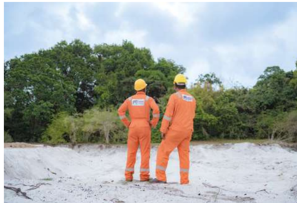
4 Once treated to within internationally compliant levels, soil is used to backfill excavated land and is covered with an ecolayer to encourage regrowth.
