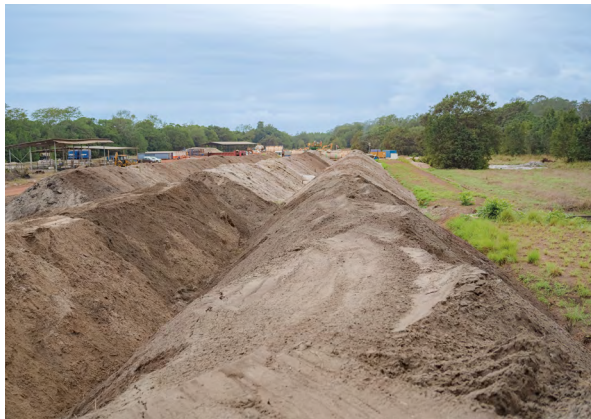
3 Treated soil is moved to lined beds to allow continuous monitoring of hydrocarbon degradation and soil quality improvement.
