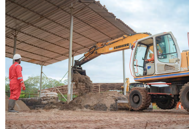
2 Nutrients are added and aerated to improve efficiency of treatment process.
